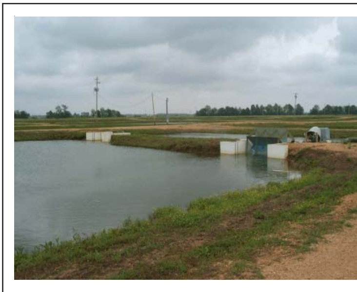
Figure 12. The split-pond system at Stoneville, Mississippi. An existing 0.32-ha earthen pond was split into a waste-treatment basin (foreground) and a fish-holding section (barely visible over the dividing levee). The two basins are hydrologically connected by a low-speed paddlewheel (at the right) and a return-flow sluiceway (at the left).
