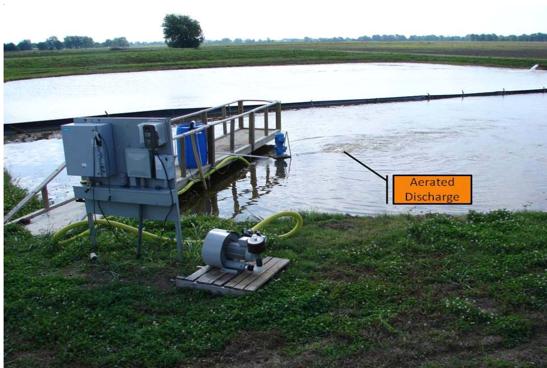
Figure 19. Prototype U-Tube with pond full. Discharge can be seen.
